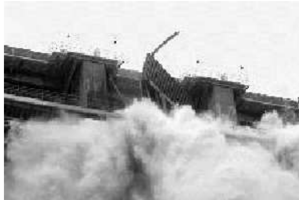
Figure 2: Failure of a spillway
