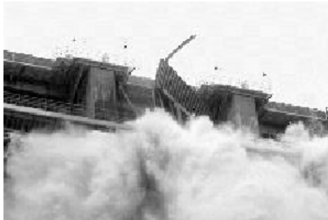
Figure 2: Failure of a spillway
